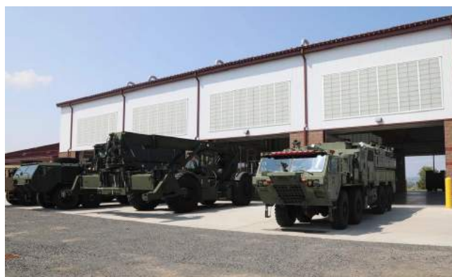
Maintenance Facilities & Hangars
